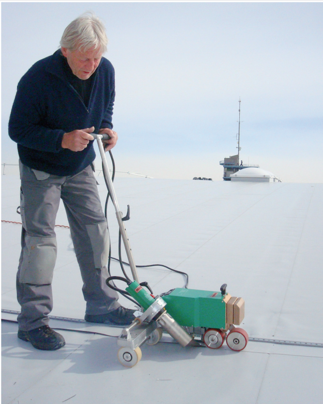
The VARIMAT V during overlap welding of the PVC strips.
