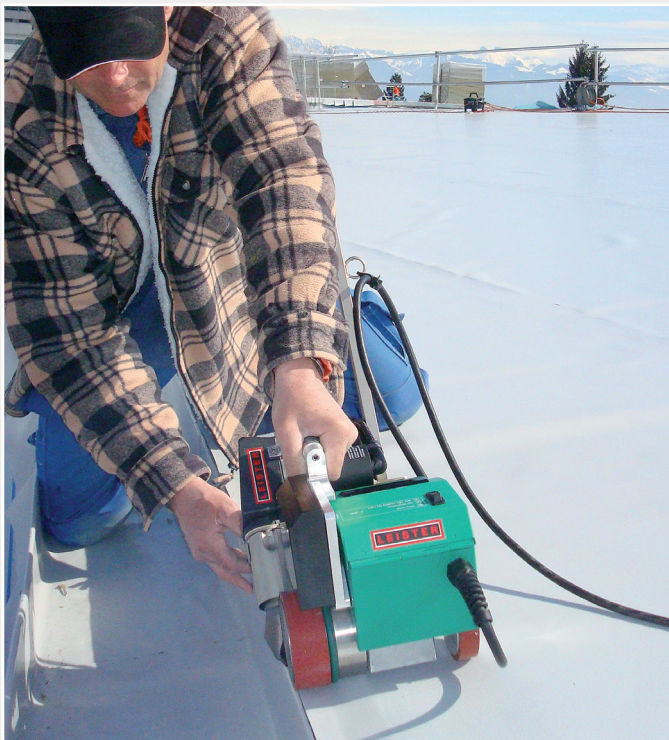
The UNIROOF E during welding of a gutter.
