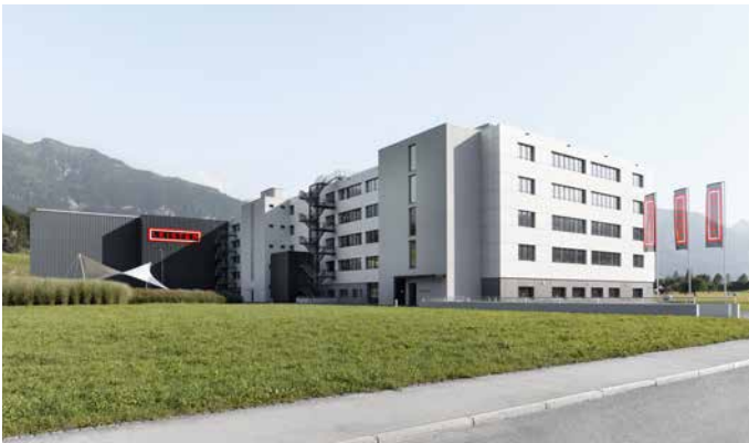
Leister Technologies AG, factory, Sarnen, Switzerland
