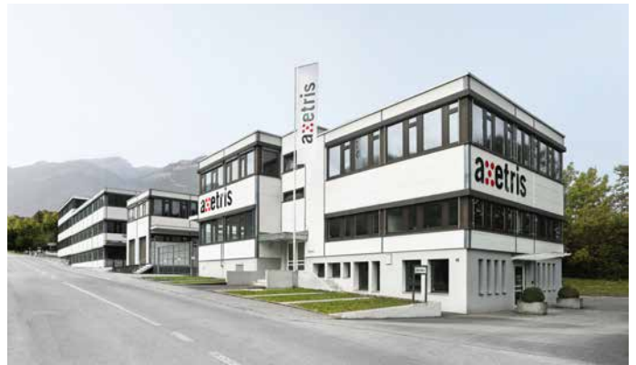
Leister Technologies AG, factory, Kaegiswil, Switzerland
