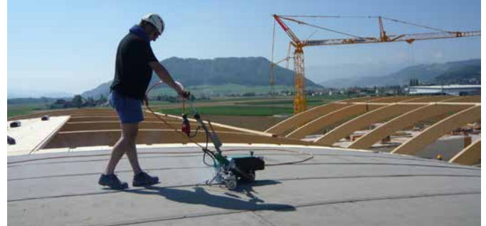
Easy unit guidance and clean working with the BITUMAT B2.
