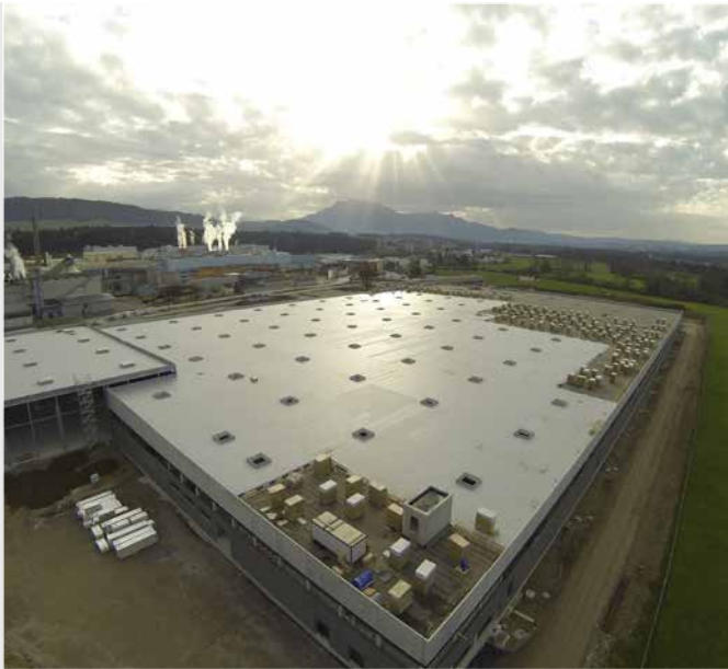
Aldi logistics center 50000m2 TPO Membrane, Switzerland
