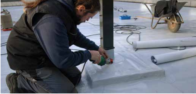
Manual welding with plastic sealing sheets.
