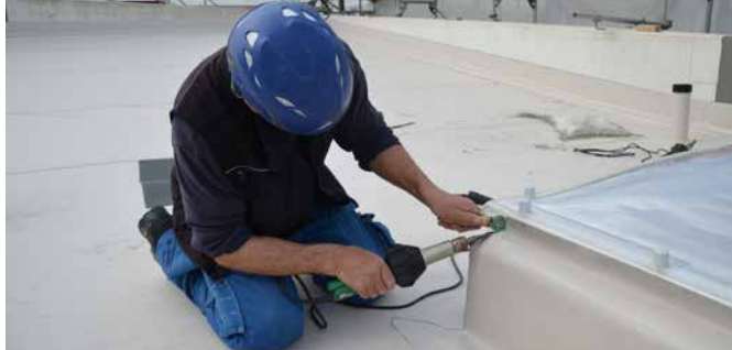
Detail work on the rooflight dome.
