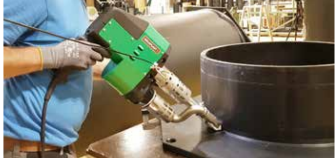
The powerful WELDPLAST S4 in use.
