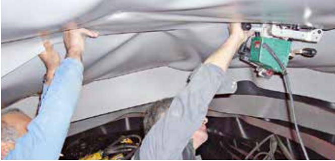
Comet operating in the tunnel ...
