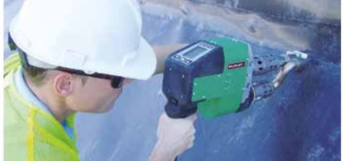
The powerful WELDPLAST S4 at work.
