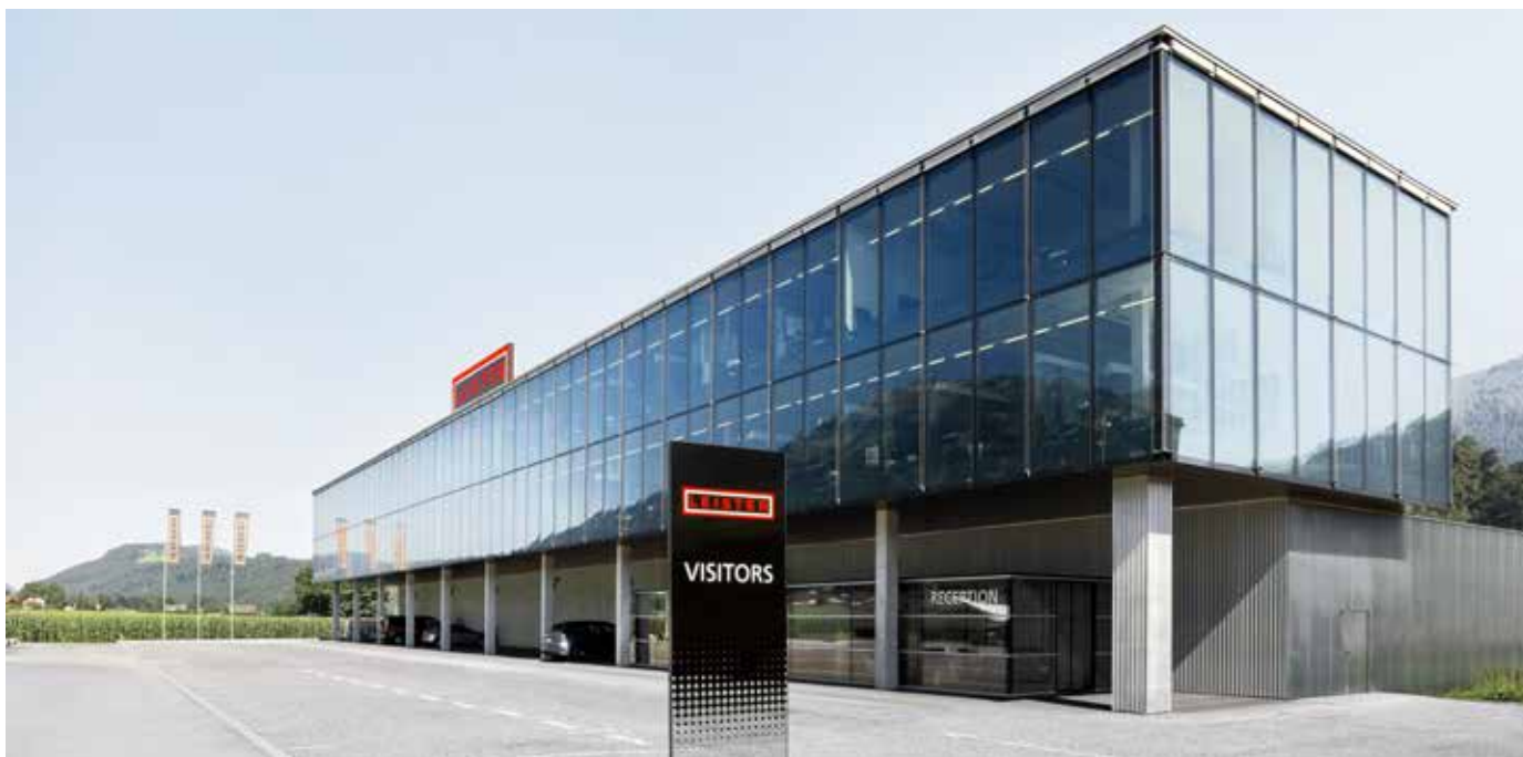
Leister AG, Headquarters, Kaegiswil, Switzerland
