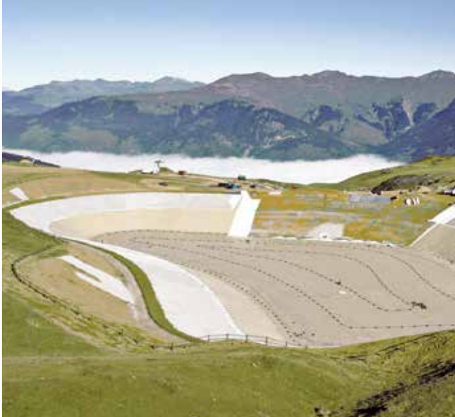
Water Reservoir, HDPE 0.08 inch (2 mm)
