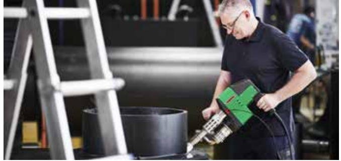
The powerful WELDPLAST S4 in use.
