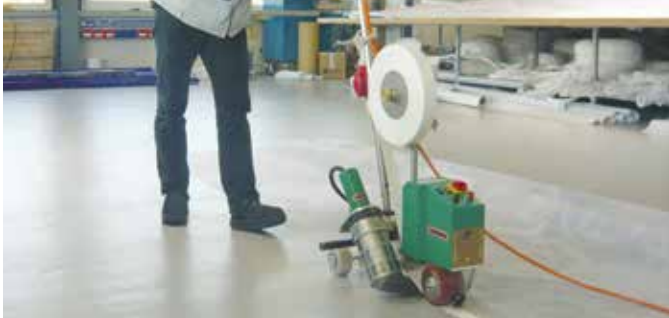
Welding tape at maximum speed.
