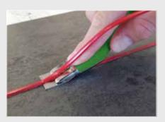
**Step 3:**Removing the excess welding rod with Quarter Moon Knife or Trimming knife.
