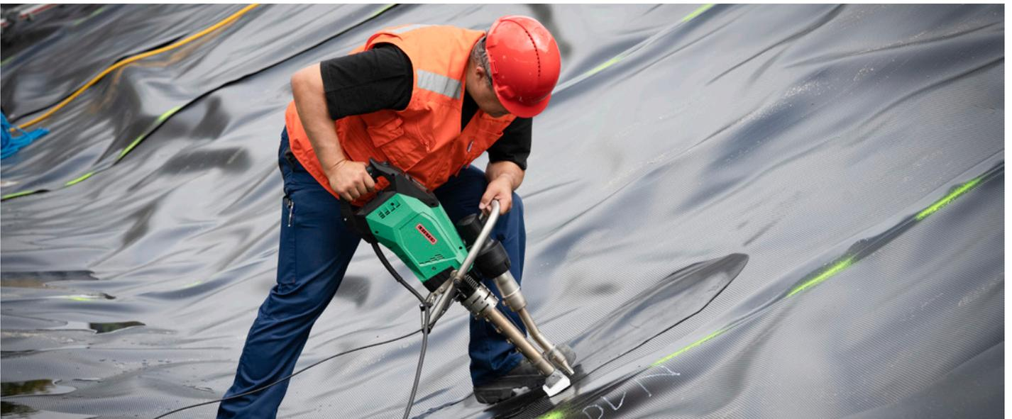
Extrusion welding of an HDPE sealing sheet with the Leister WELDPLAST 605 extruder in a pond
